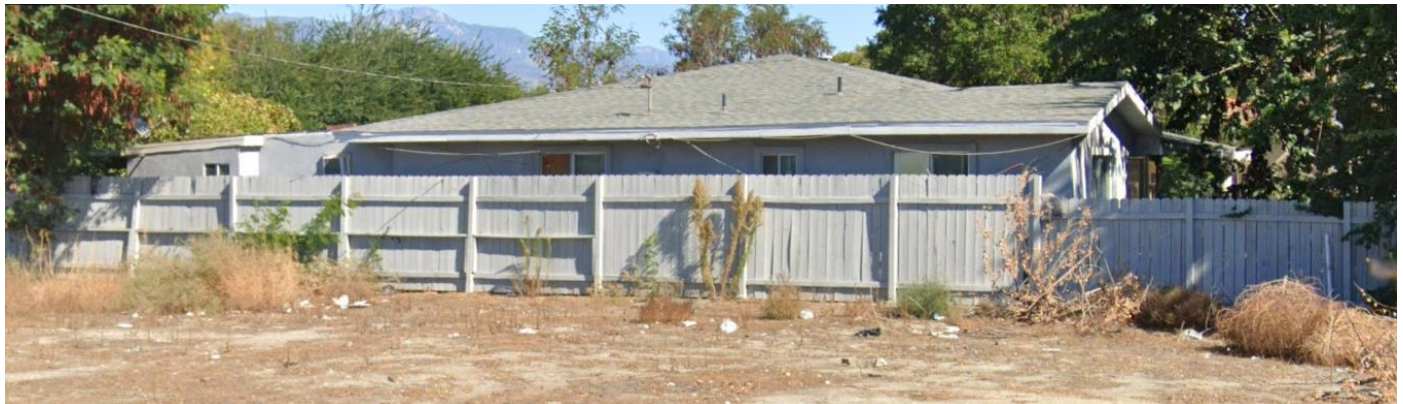
Residence Overview (View NE)
